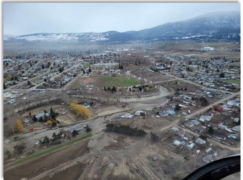
Aerial view of Pine Street and Coldwater River avulsion after the river was moved back to its original channel.
