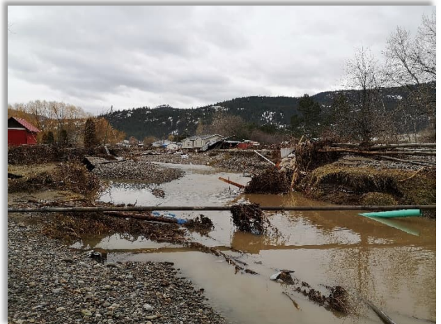
FortisBC gas main supplying entire City of Merritt exposed in Coldwater River avulsion channel.
