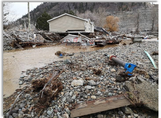
Road damage, exposed and damaged utilities, and property damage along Pine Street.
