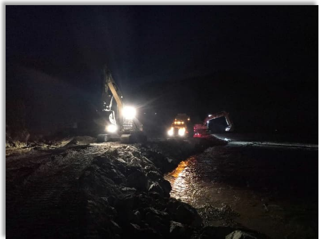
Emergency response activities included construction works extending beyond normal hours.
