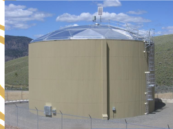
South East Balancing Reservoir
