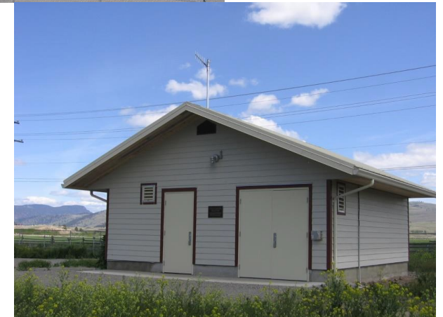
Kengard Pump House
